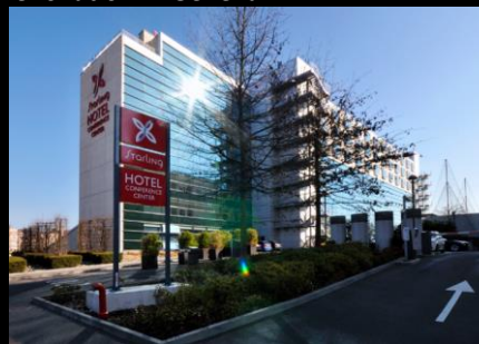
EPC solution for the private service sector: a hotel renovation in Geneva
