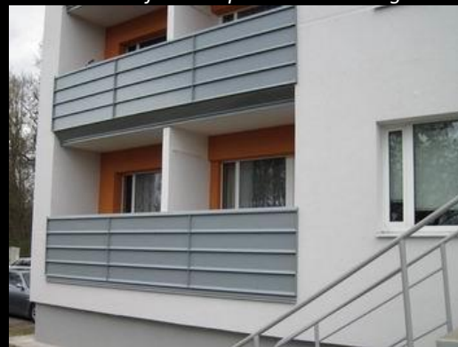
EPC renovation of multi-apartment buildings
